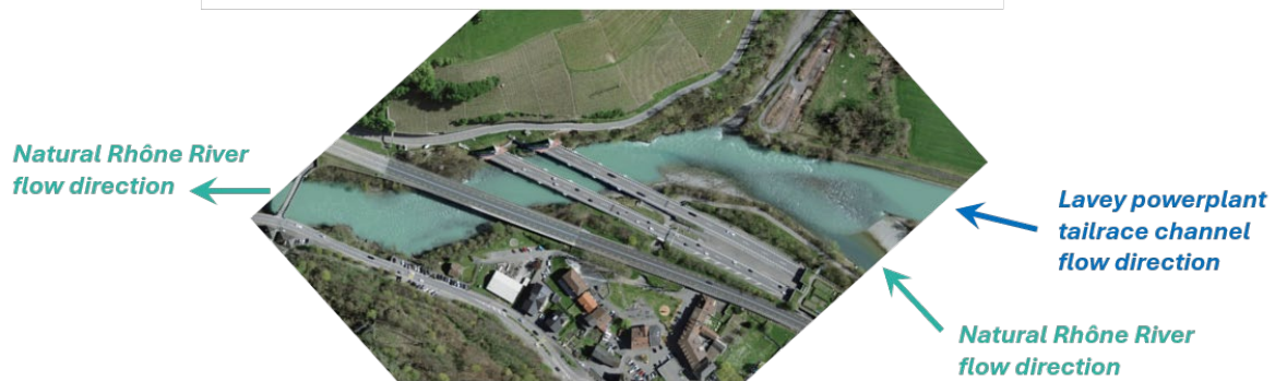
Figure 32. Zoom on the high velocity values observed at km ~143 from Figure 30 . Confluence between the natural Rhône River and the tailrace channel of Lavey powerplant.
