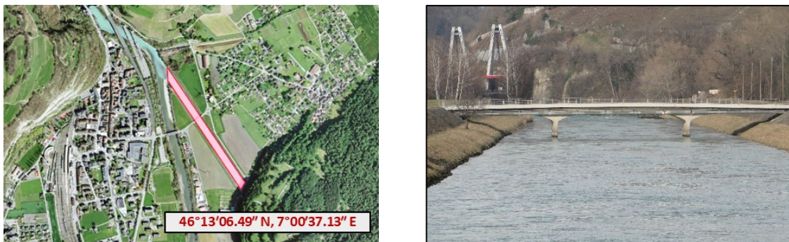
Figure 42. Geographic location and photograph of the Lavey hydropower plant tailrace channel considered for the hydrokinetic potential evaluation.
